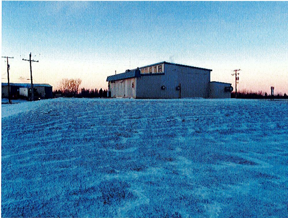
Water Treatment Plant Building, Underground Reservoir in Foreground
