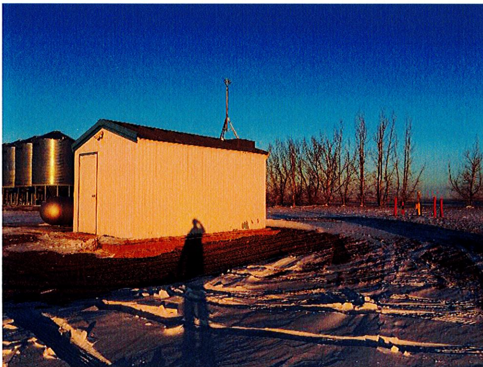
Well #3 Controls Housing
