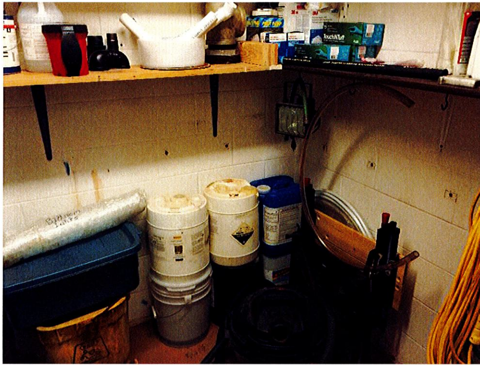
Plant Storage Room
