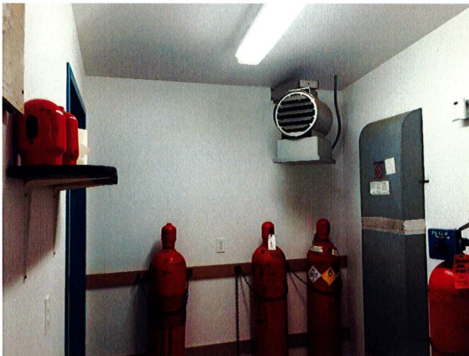
Separated Chemical Room
